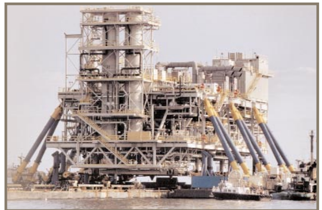
Fig. 4. Setting the topside in place.
