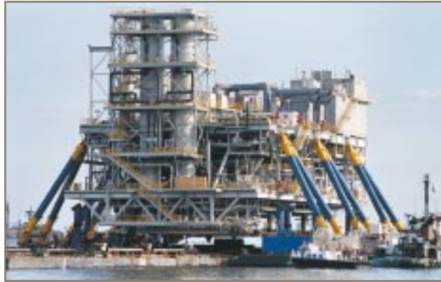
Versatruss's new lifting system installing a Chevron platform.
