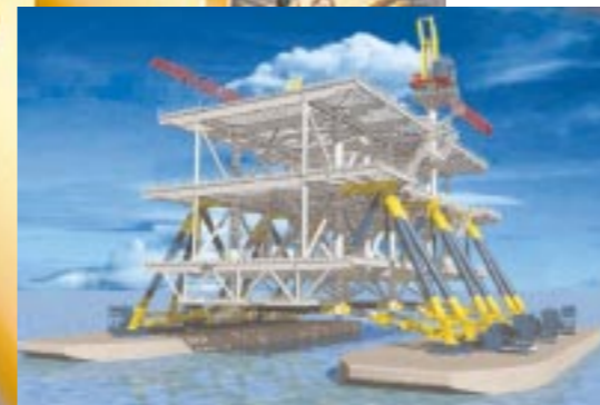
ABOVE: The two 55m long Versatruss lift barge were each kitted out with four custom-made booms. Base of each boom is secured to the lift barge centreline using a spreader beam.
